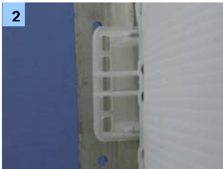
2 Position the curved section of the signAclip against the fin with the predrilled holes
