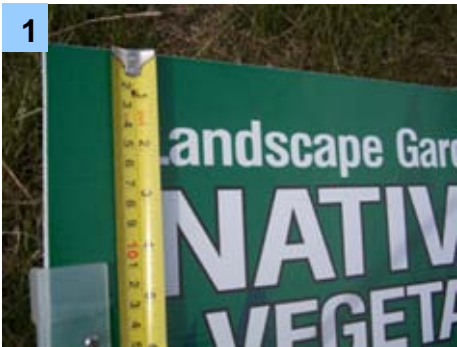
1 Positioning signAclips Fit each signAclip at the same measured distance (minimum of 100mm) from the top of your panel sign.
